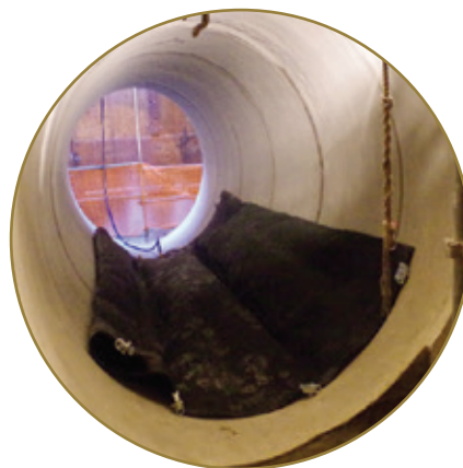
Placing – pillow plug should be positioned horizontally
