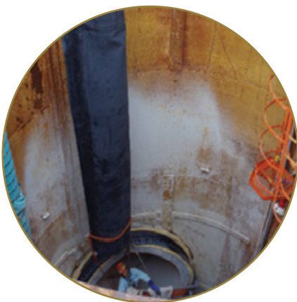
Inserting a folded pillow plug
